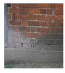
Ordnance Survey Bench Marks are marks made by Ordnance Survey to record height above Ordnance Datum. If the exact height of one Bench Mark is known, the exact height of the next can be found by measuring the difference in heights, through a process of spirit levelling.
